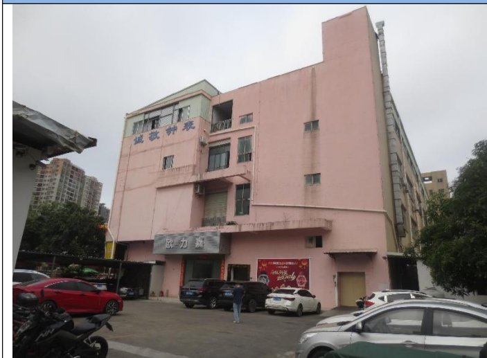
Factory building view
