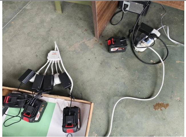
Battery charge check-10:03
