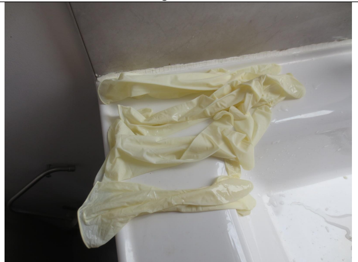
Leakage test view
