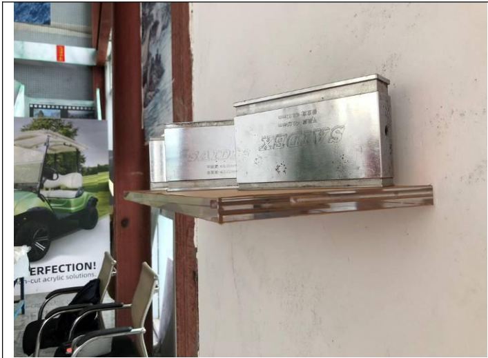
Static loading test
