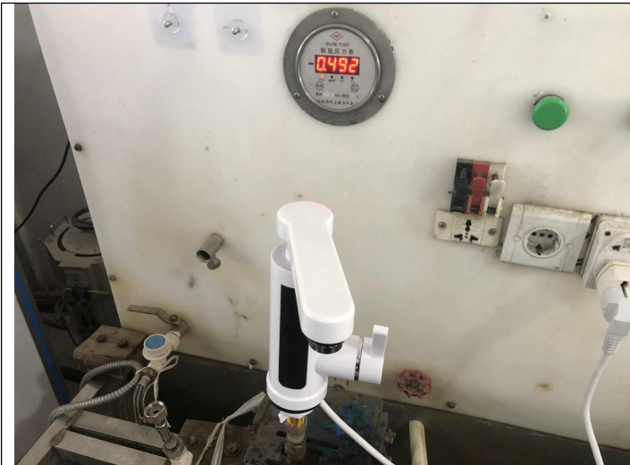
Water pressure check
