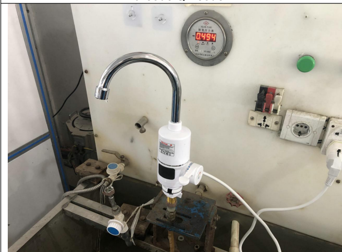
Water pressure check
