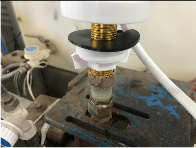
Assembly/ installation check
