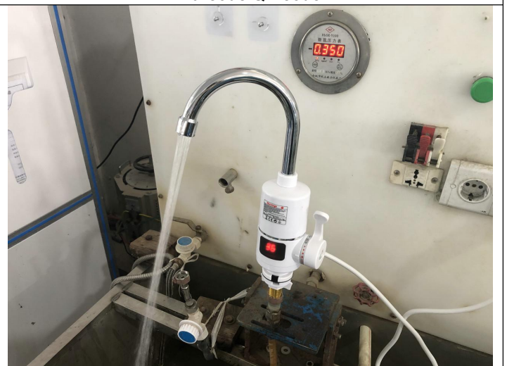
Water pressure check
