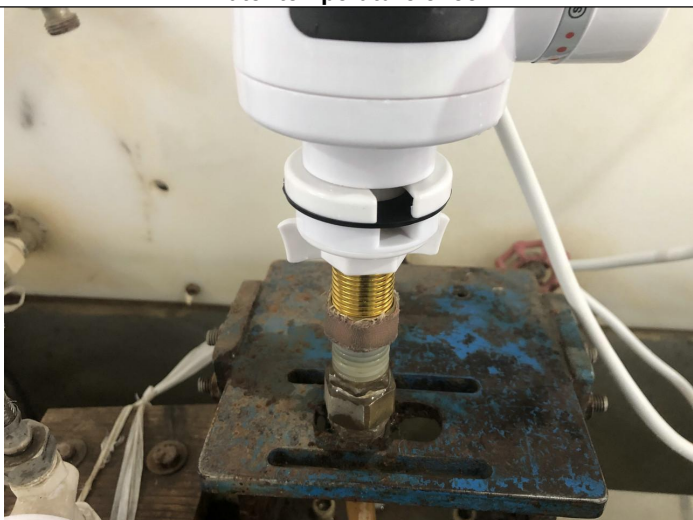
Assembly/ installation check
