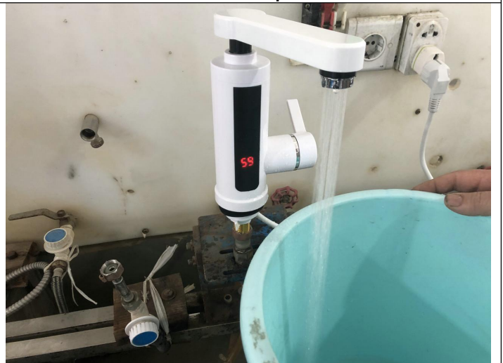
Water flow inspection
