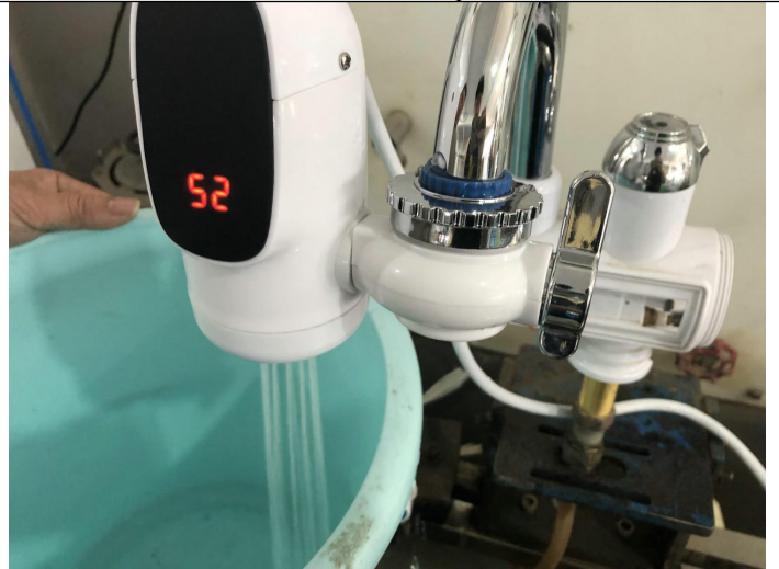
Water flow inspection
