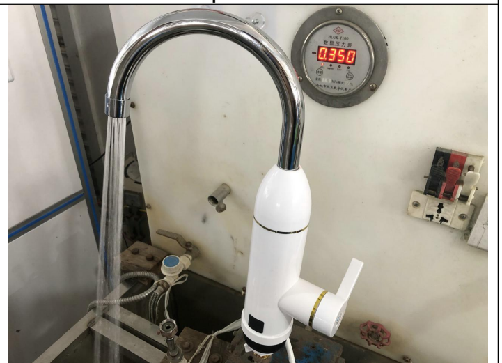
Water pressure check
