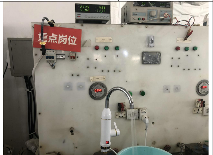
Water flow inspection
