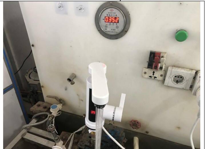
Water pressure check
